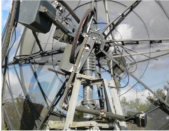
(Fig.1) 4.4m TVRO dish, a product of Paraclipse, at JH1KRC has no construction that fits for detecting the elevation angle directly at the elevation rotary axis.
